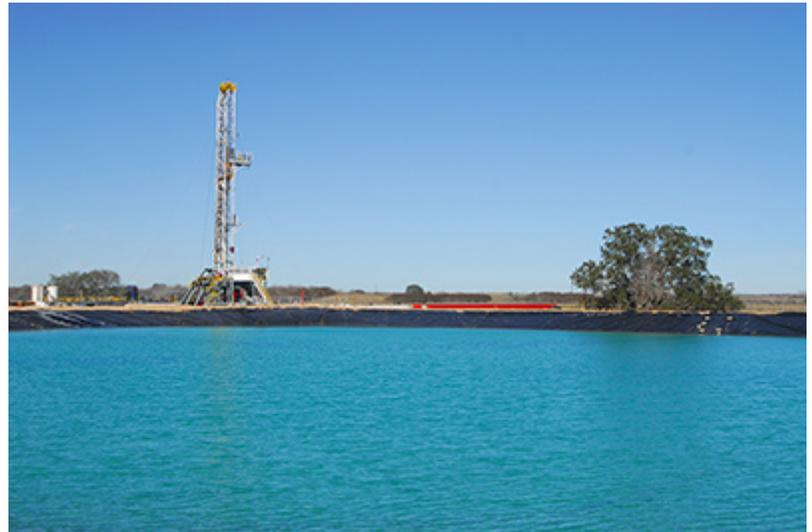
Pioneer Water Management, LLC is utilizing lined, engineered water storage ponds for improved water conservation efforts, storage capacity and distribution efficiencies. Here, a drilling rig is behind the lined containment berm of a water storage pond.
