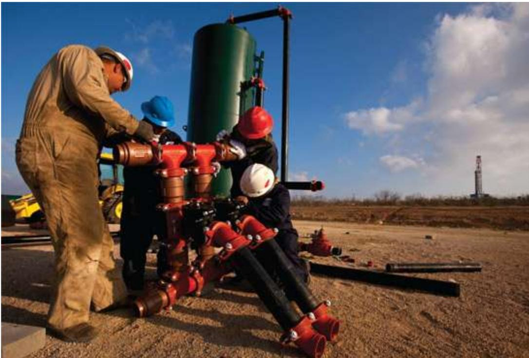
Fisher Lease Services workers construct the free-water knockout for a tank battery downhill of Patterson-UTI Rig #208 drilling for Pioneer near Rankin, Texas.
